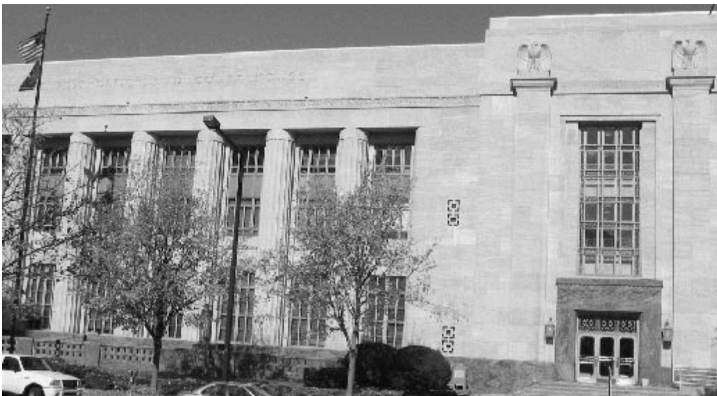
Historic Post Office Building in Knoxville
